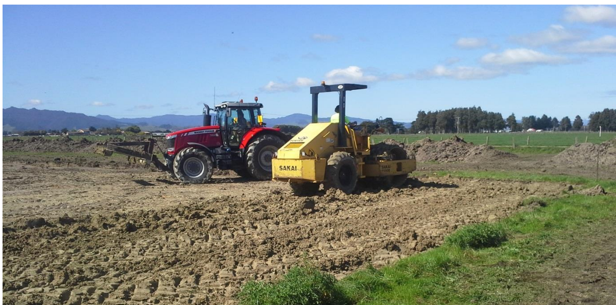
Figure 6.1: Trial Compaction Area Preparation
