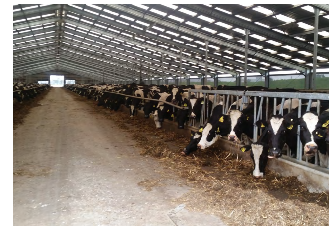
It is possible to install a few locking yokes at the end of the feed face to provide a cow handling area. Alternatively consider including a vet race in the building design.
